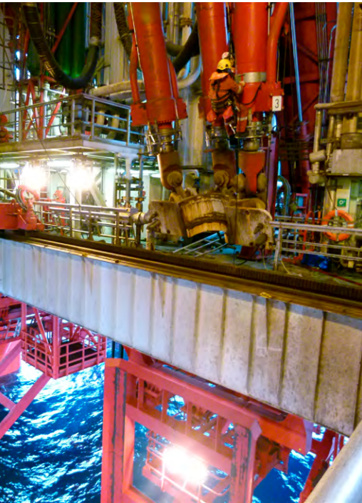
Riser Fatigue mounting of sensor
